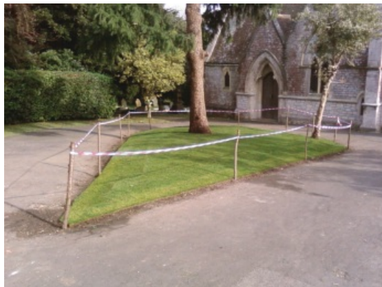
The area in front of the Chapel after turf laying
