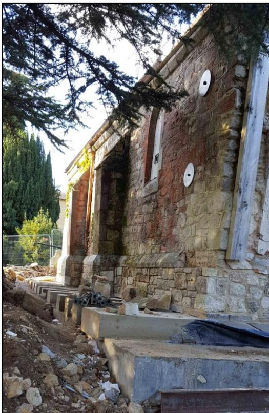
The exposed beams and some of new stonework at the bottom of the south (rear) elevation of the West Chapel
