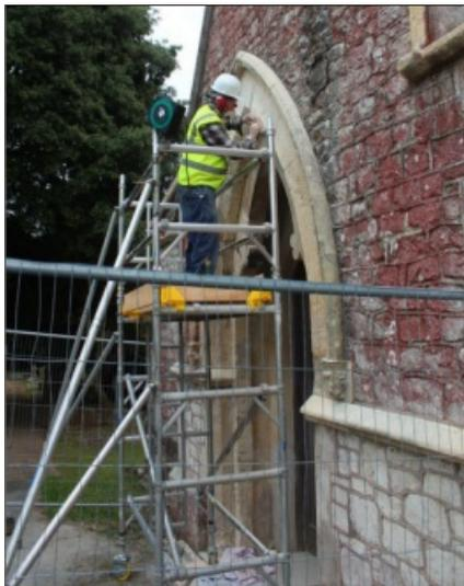
But the most visible activity has been the restoration of the stonework around the main doorway arch, which was in a very poor state of repair - and the oak doors themselves.
